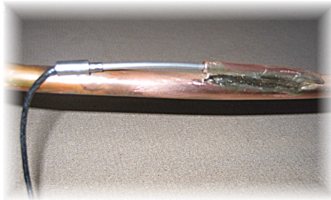
Diagram 16. Remote sensor silver soldered to refrigeration line.
